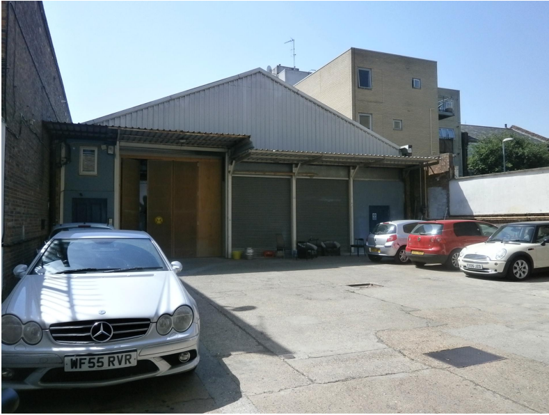
Existing warehouse building
